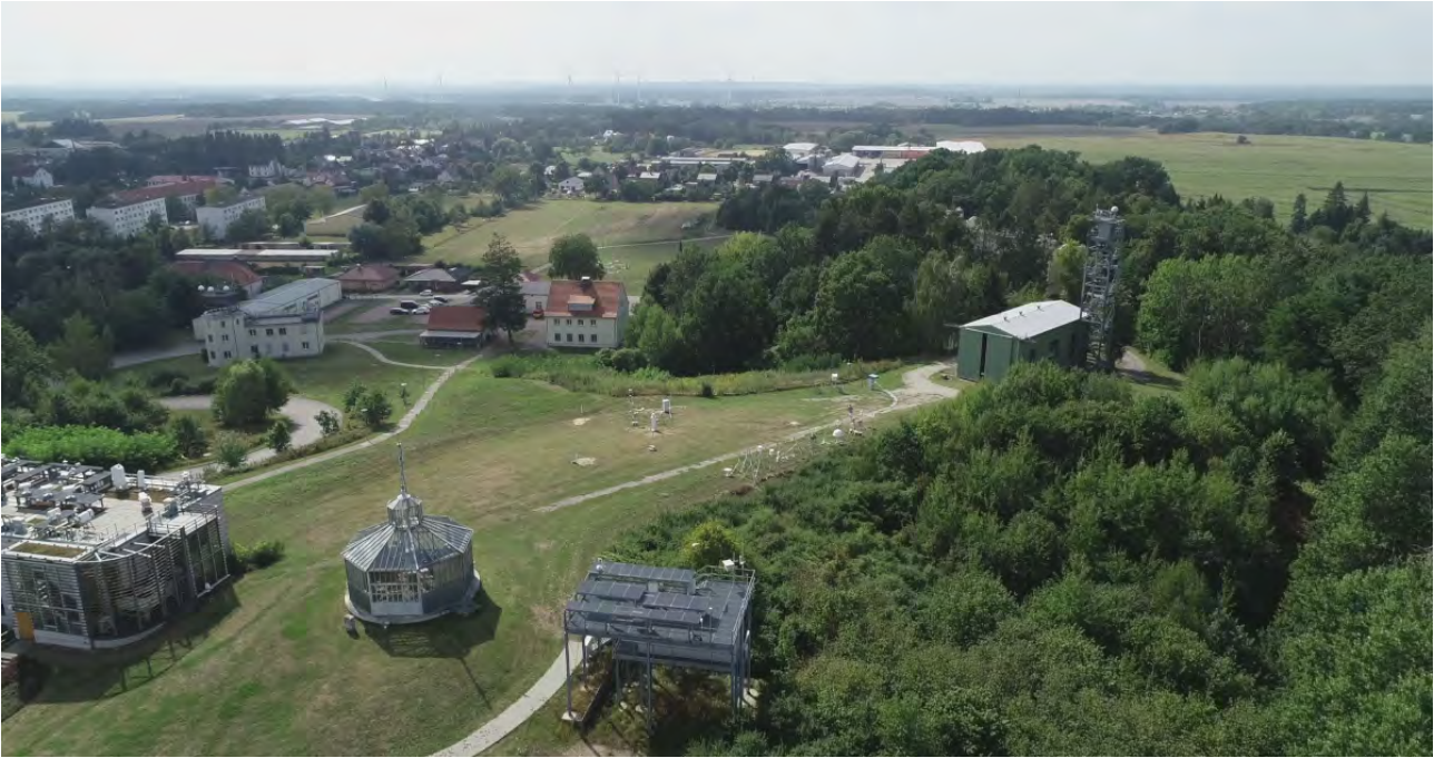
Figure 4.5: Aerial view of the observatory site towards southwest at the time of the campaign.
