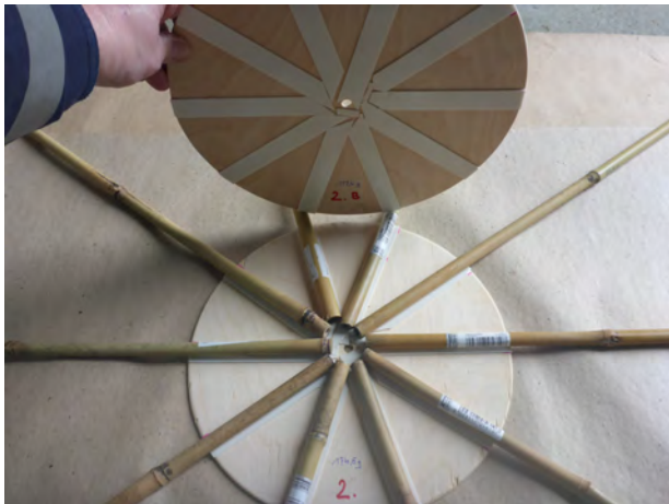
(c) Align the second plate of plywood
