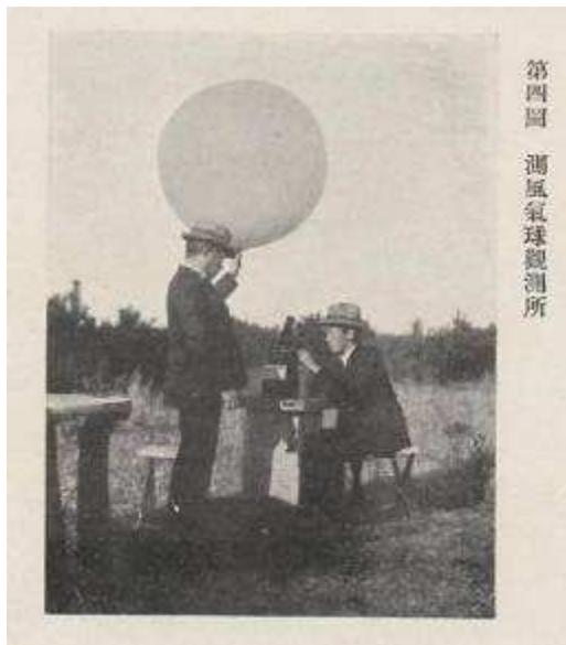
Pilot balloon and theodolite on a base
